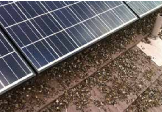
The Problem - Pigeon droppings accumulate on roofs under solar arrays.
