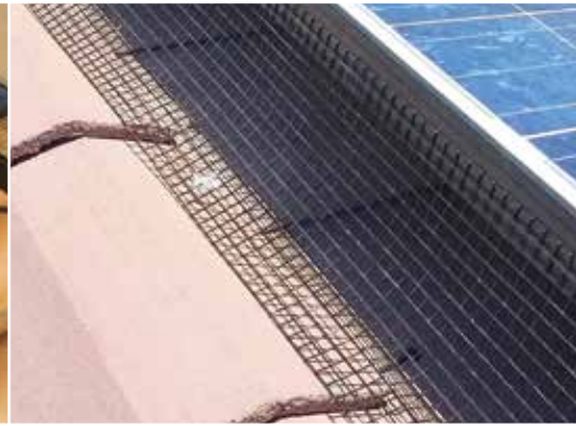
The mesh is secured on all sides, permanently excluding birds and other wildlife.
