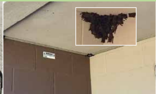
A single row of Bird-Shock at the top of this wall eliminated a bat infestation.
