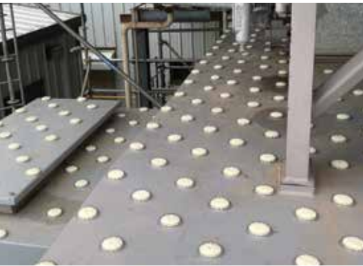
A large flat surface at an industrial site is protected with Optical Gel spaced at 6 inches.
